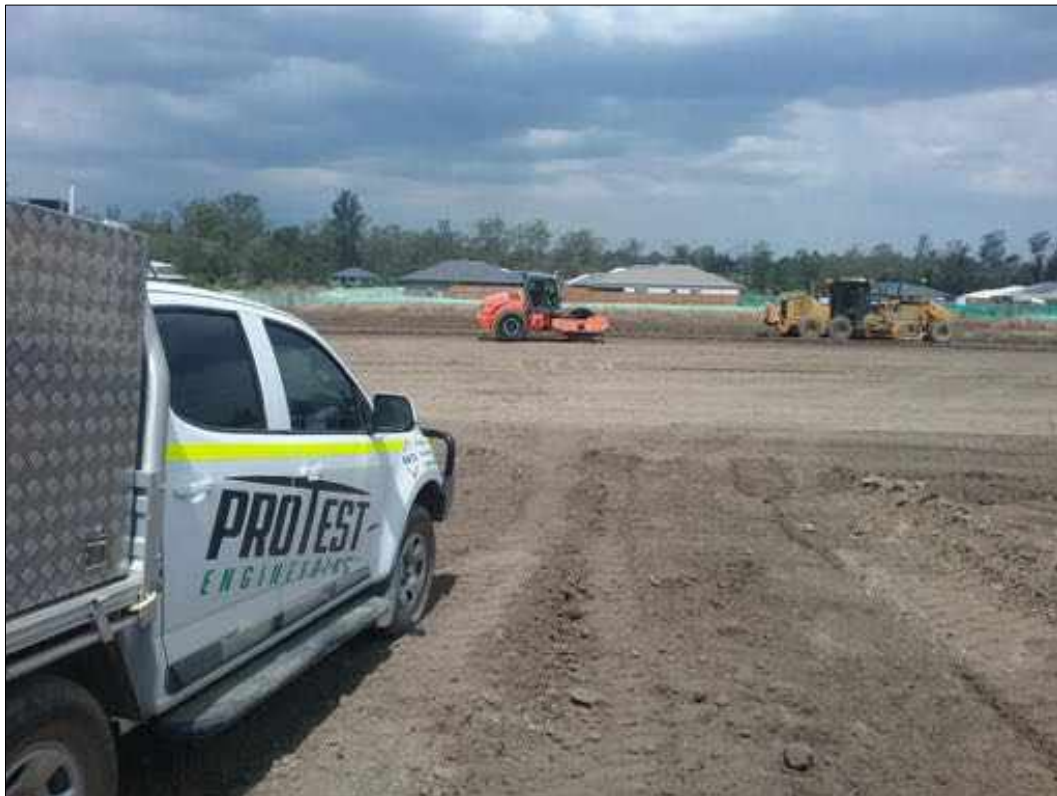
Figure 4 – Pad foot roller and grader used to trim and compact placed fill materials. (Taken 11 October 2019)
