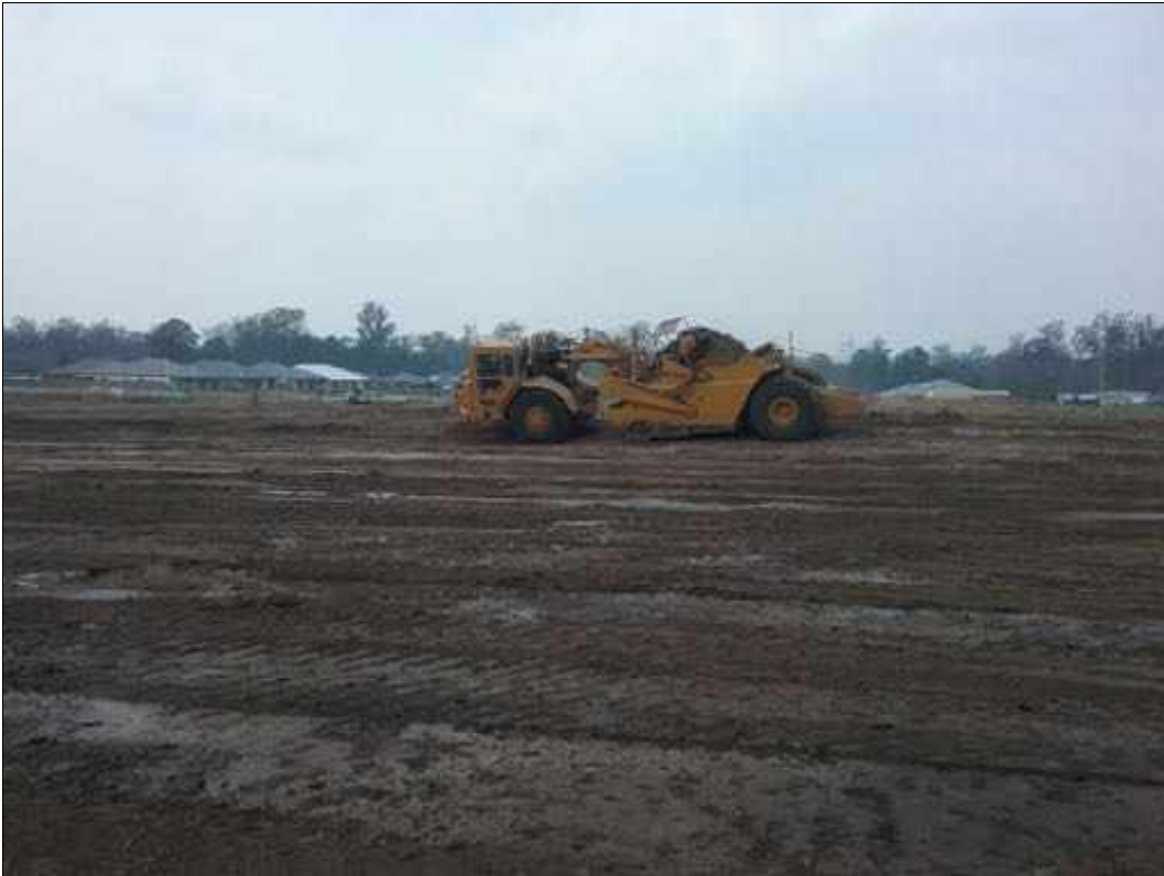
Figure 1 – Topsoil strip and removal of organic/unsuitable material across the site area using the 623G Scraper. (Taken 8 October 2019)
