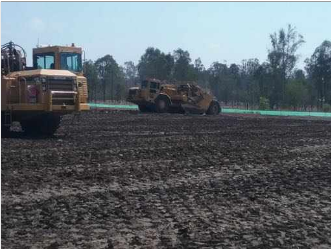
Figure 2 – 623G Scrapers used throughout bulk earthworks component to spread and place fill. (Taken 10 October 2019)
