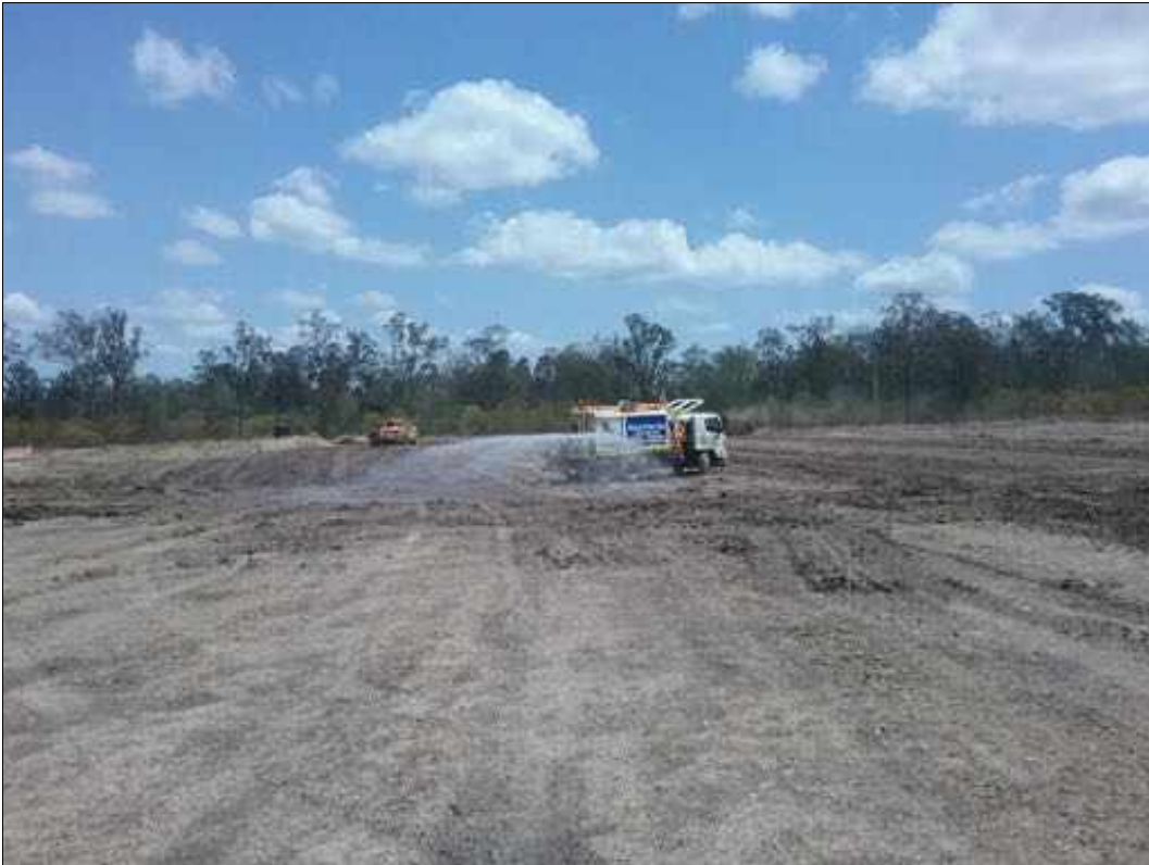
Figure 3 – Water cart used during the bulk earthworks component to moisture condition fill prior and during placement. (Taken 11 October 2019)
